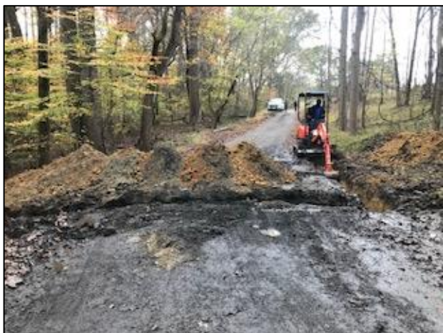
(above) Pops Christian digs a trench on the up-hill side of the road that will feed the cross-road trench. (below) Alan Goodman brings a load of asphalt millings to the scene in the Gator, for spreading on the road. (top right) Pops inspects the gravel-filled trench prior to back-filling. Photos by Alwin Alleyne.
