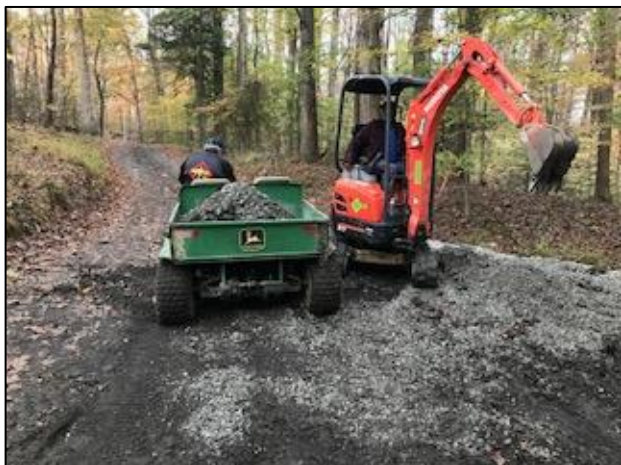
(above) Pops Christian digs a trench on the up-hill side of the road that will feed the cross-road trench. (below) Alan Goodman brings a load of asphalt millings to the scene in the Gator, for spreading on the road. (top right) Pops inspects the gravel-filled trench prior to back-filling. Photos by Alwin Alleyne.
